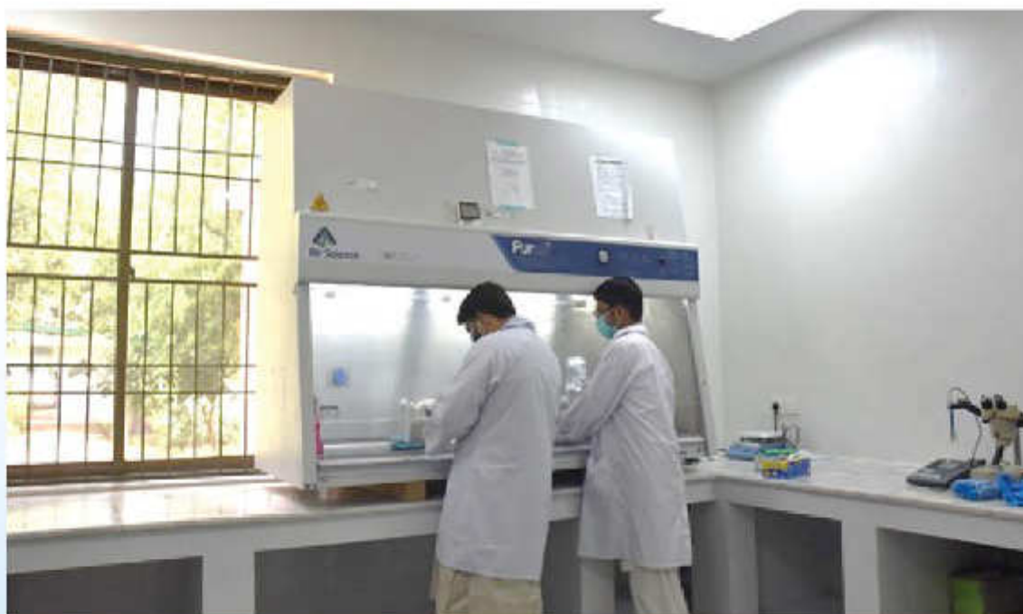
Renovation of Mycoplasma Section
