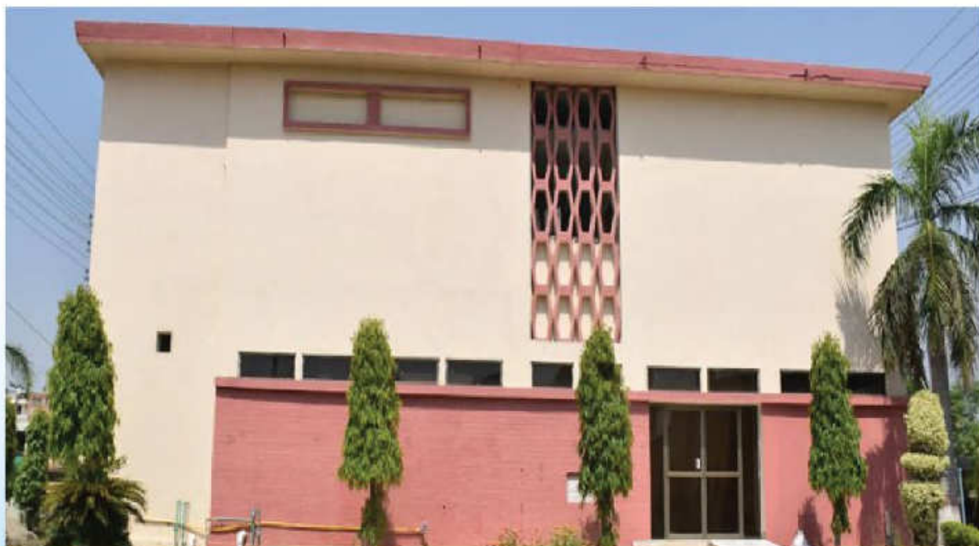
Renovation of Cell Culture Section Building
