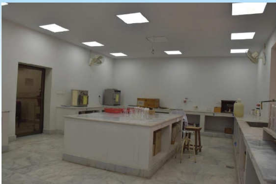
Renovation of Media Preparation Room
