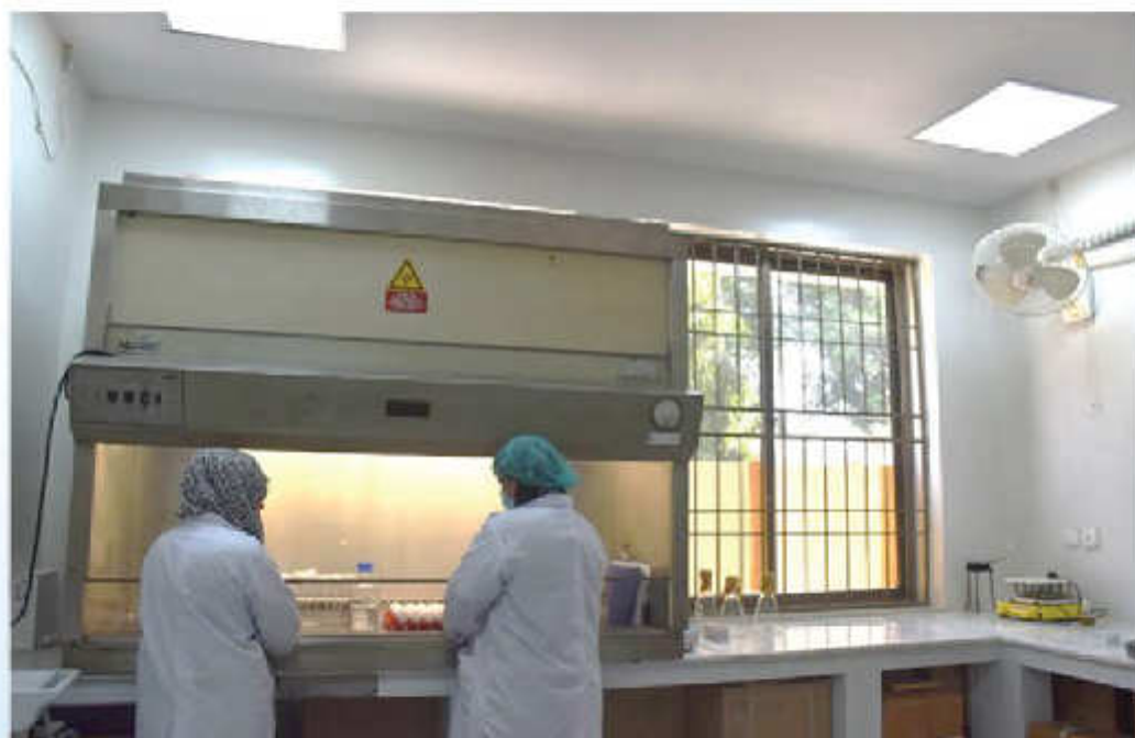
Renovation of NDV Section Lab
